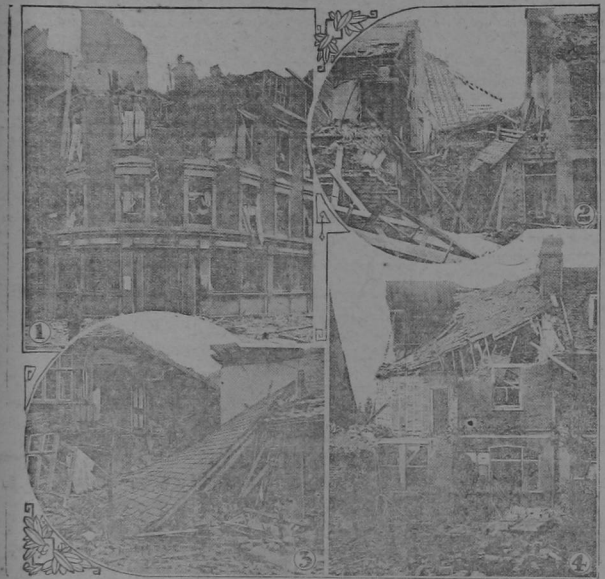
These pictures of the damages caused to houses in London by the recent Zeppelin raid show: 1, bank in London damaged by bomb; 2, house splintered by explosion; 3, another view of the same house; 4, damage to brick dwelling caused by bomb which crashed through roof and exploded inside the house. Especial attention is called to the fact that the signs on the bank in No. 1 are obliterated—obviously by order of the censor, in order to keep information of the location of the damage from the Germans.
